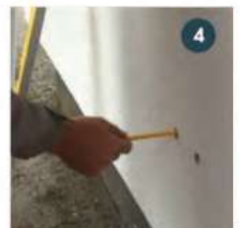
Measure depth to substructure
