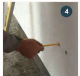
Measure depth to substructure
