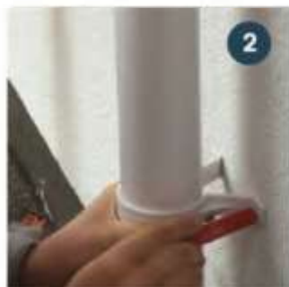
Mark the wall
