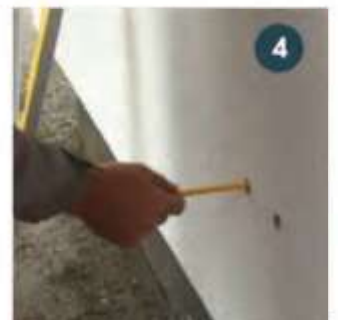
Measure depth to substructure
